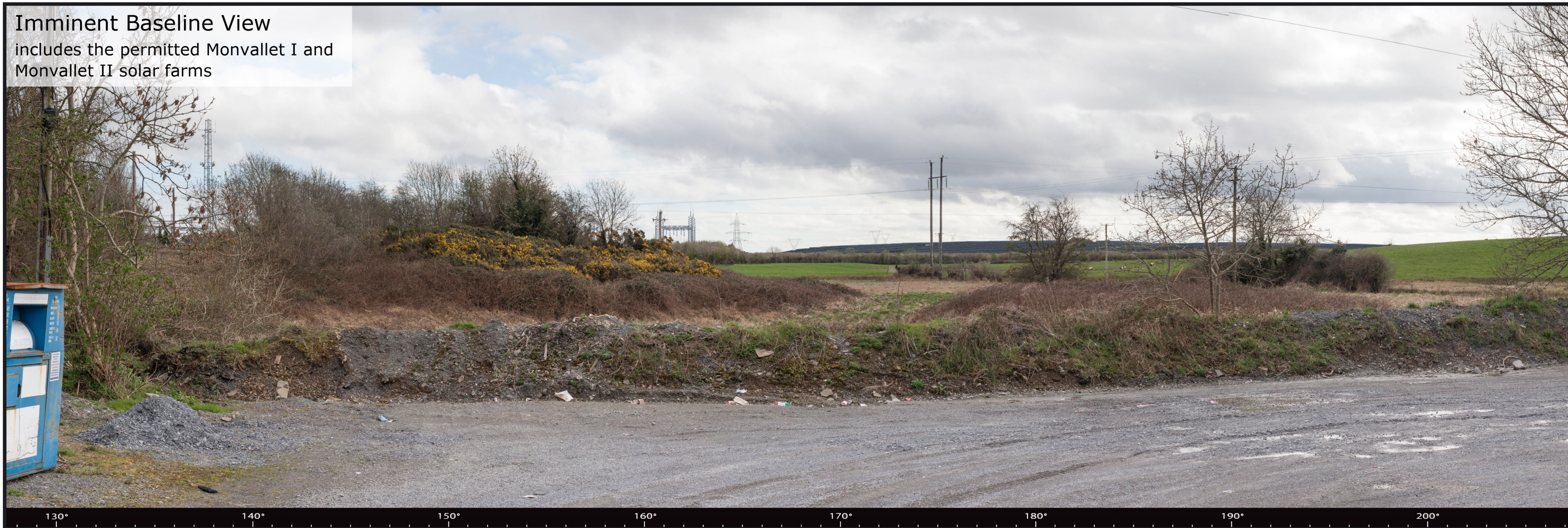
Outline View indicating physical position and scale of the proposed substation irrespective of screening
